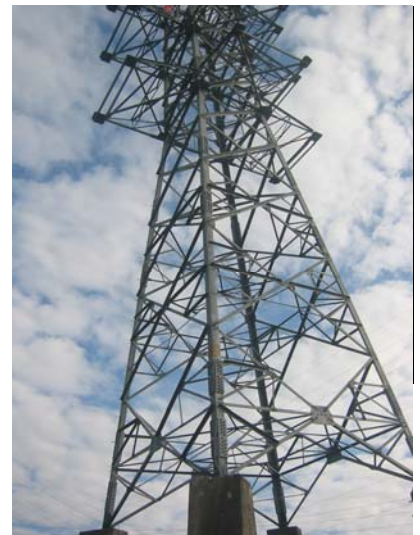
An electric tower that moved during an earthquake—but no longer works.. It now stands as a memorial .
